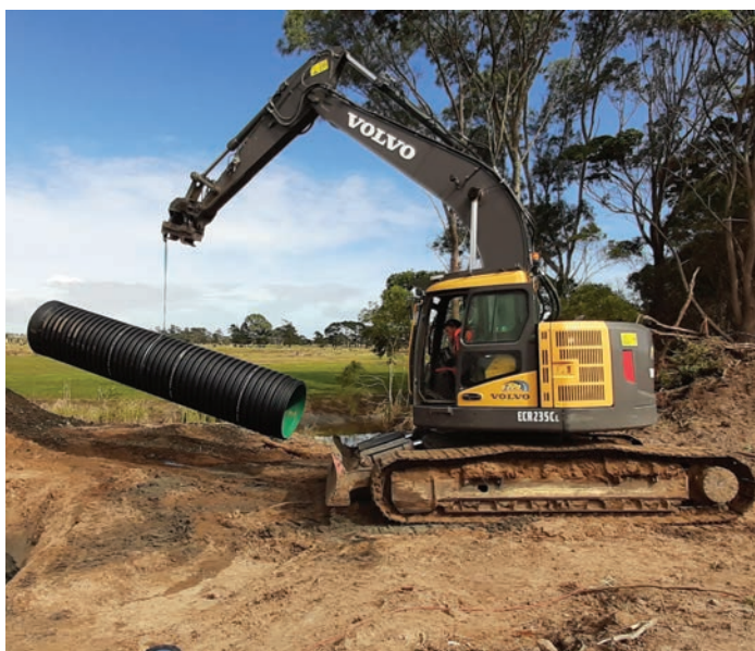
EUROFLO® rural pipe being installed on farm
