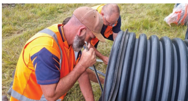
Onsite installation of rubber rings.
