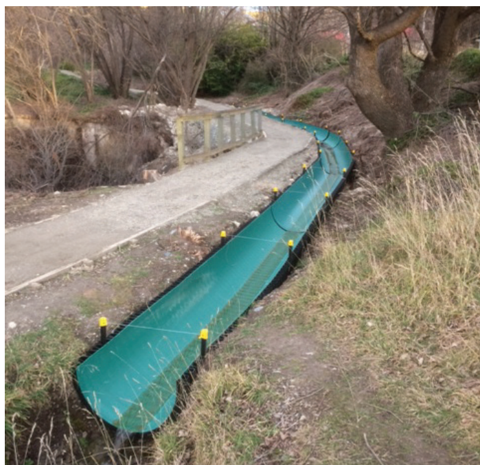
EUROFLO® fluming as seen on the St Bathans cycleway
