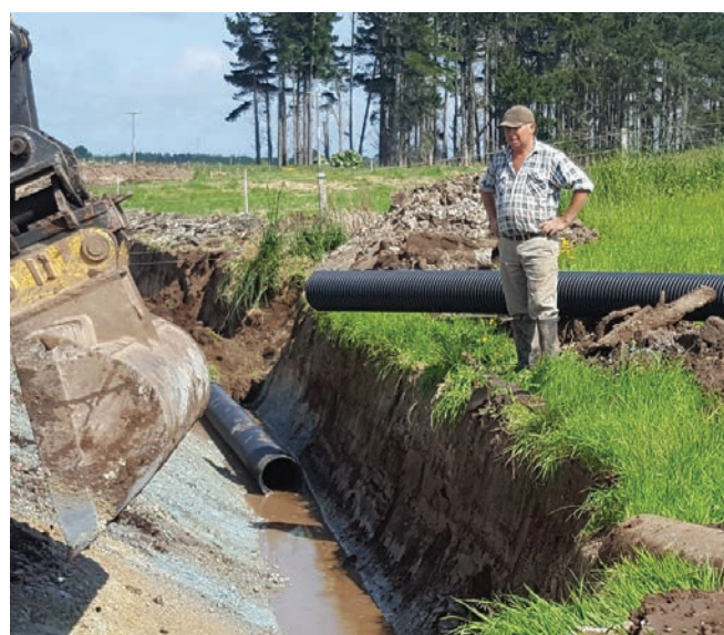
Slotted pipe being installed on farm
