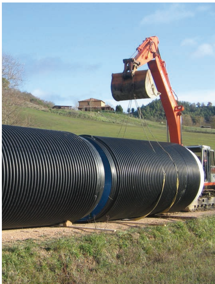
EUROFLO® large diameter being installed on farm
