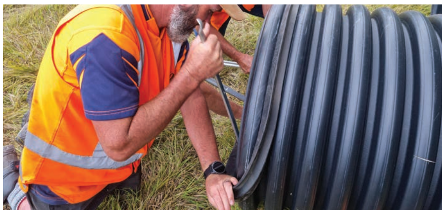
Onsite installation of rubber rings
