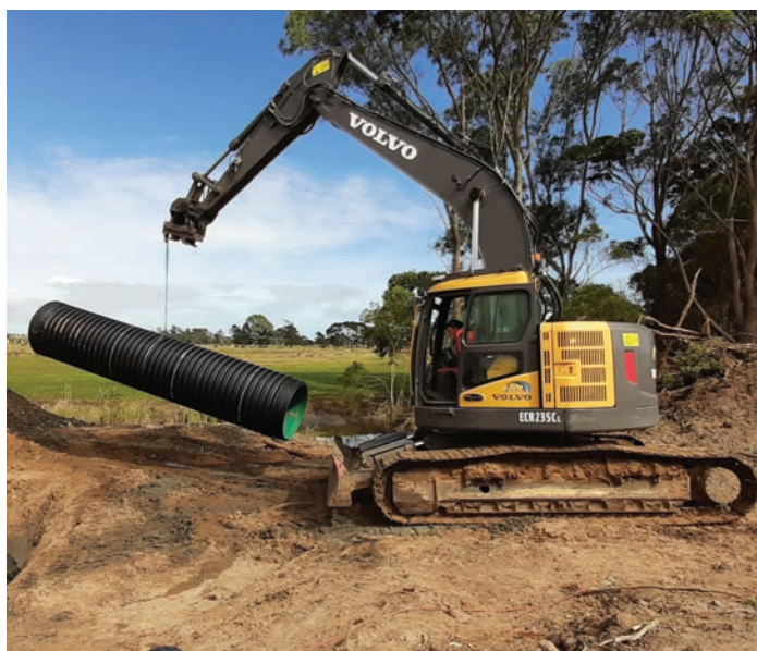
EUROFLO® rural pipe being installed on farm
