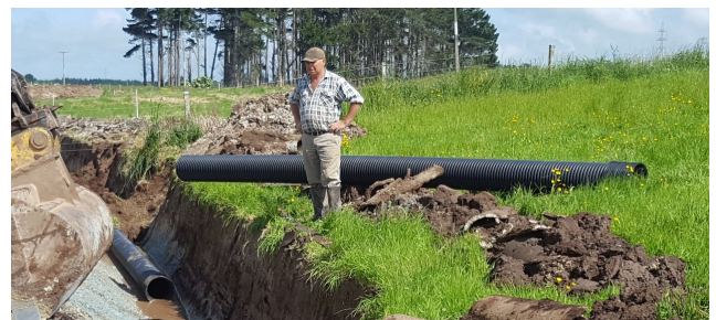
Slotted pipe being installed on farm
