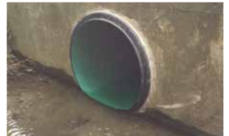
Installed EUROFLO® in headwall
