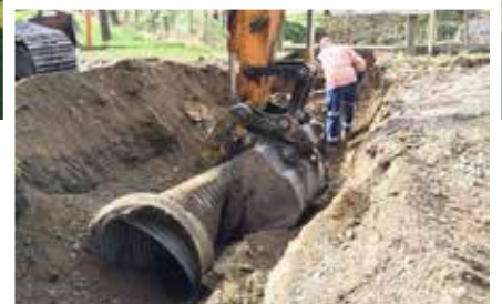
Removal of old corrugated steel pipe
