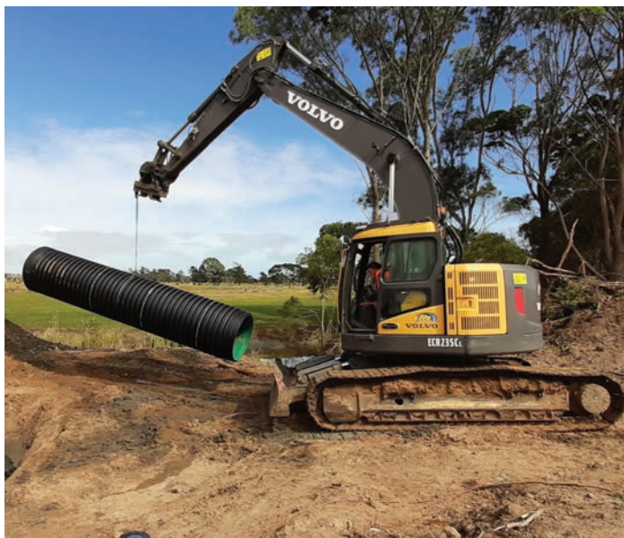
EUROFLO® rural pipe being installed on farm
