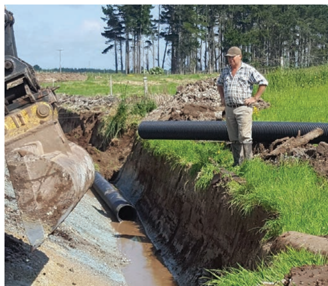
Slotted pipe being installed on farm
