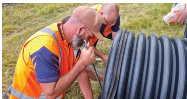
Onsite installation of rubber rings.
