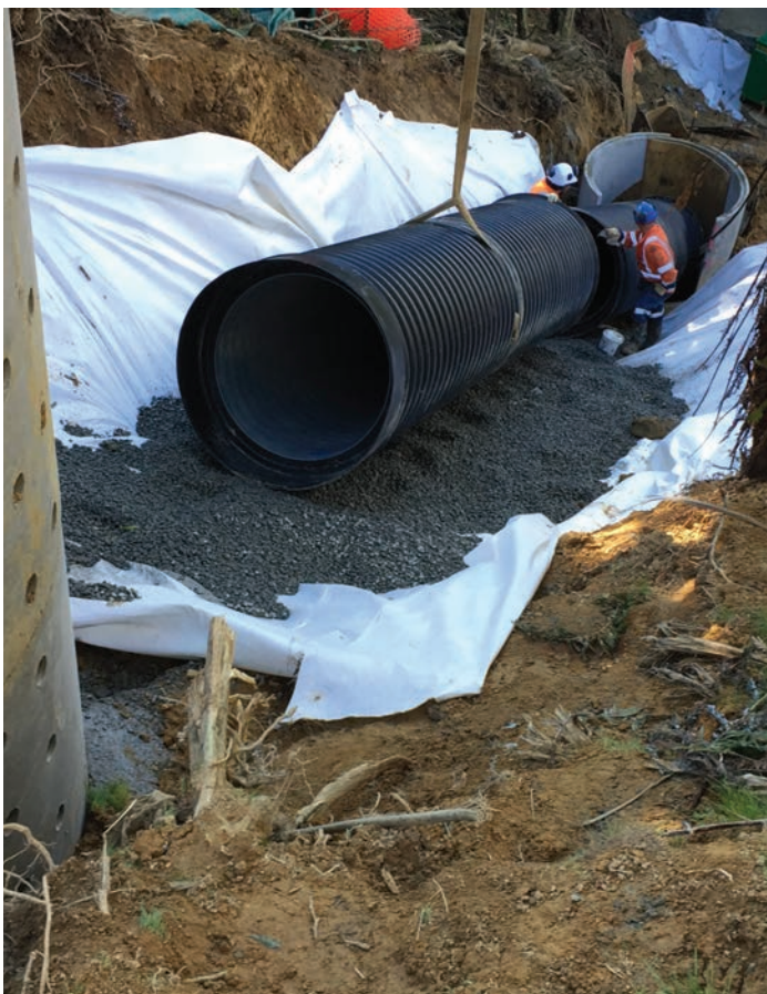
Civil SN8 pipe being laid down a hillside in Wellington.
